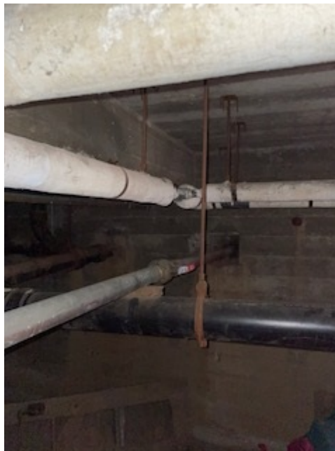
Asbestos-containing TSI in Girls Locker Room Crawlspace
