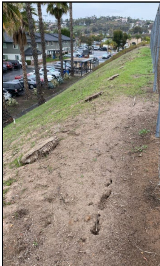
Movement of Old Fence Footings (Viewed to the North)
