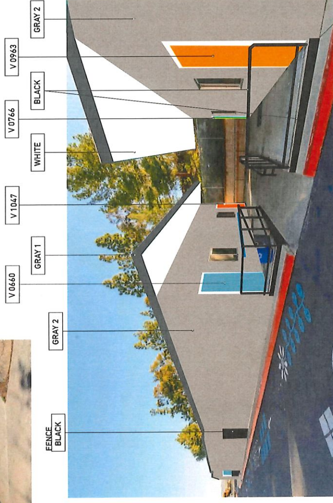
P1-P5 PRIMARY FIELD COLOR: GRAY 2 ALL FASCIA: GRAY 1 ALL UNDER EAVES: WHITE ALL NON-ALUMINUM PAINTED WINDOW FRAMES: WHITE ALL BACKPACK HOOK BOARDS: V 0640 ALL RAILINGS/BASES: BLACK ALL GATES/FENCES: BLACK ALL UTILITY/STORAGE DOORS: V 0619 CLASSROOM DOORS ALTERNATE: (V 0766), (V 0943), (V 0640), (V 1047)
