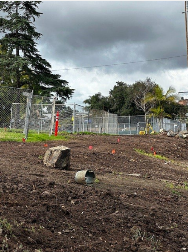
Rancho Elementary Slope Drainage Improvements
