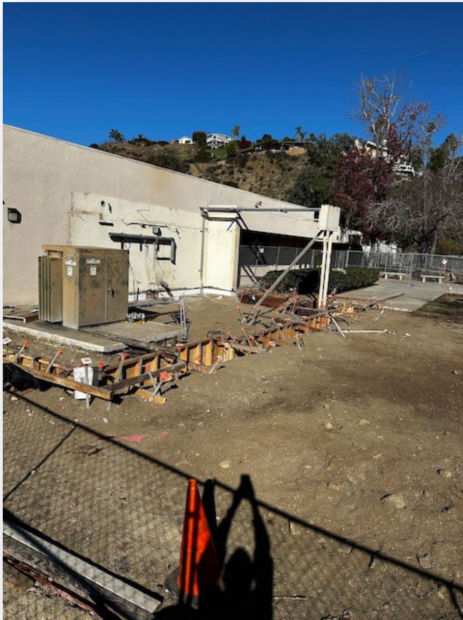
Demo Existing Tower Enclosure
