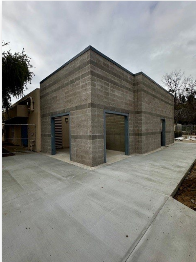
New Cooling Tower Enclosure
