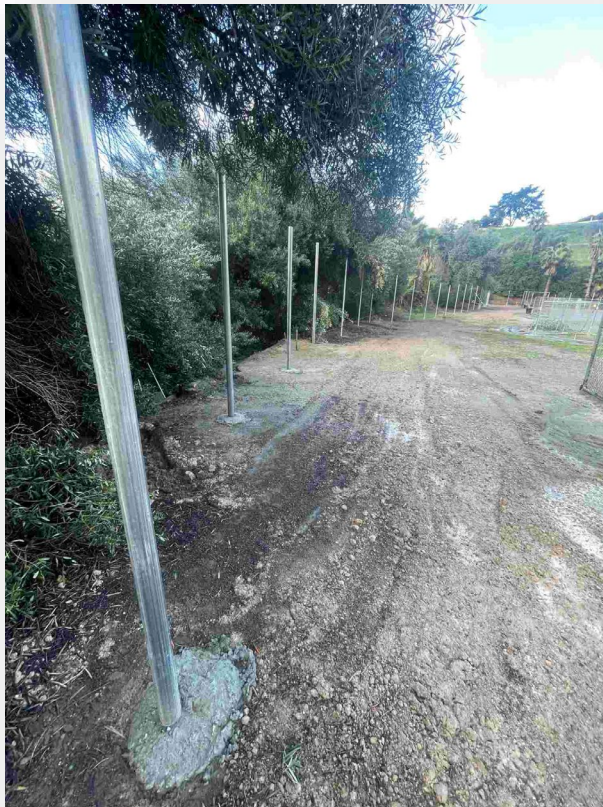
Avondale Elementary Security Fencing
